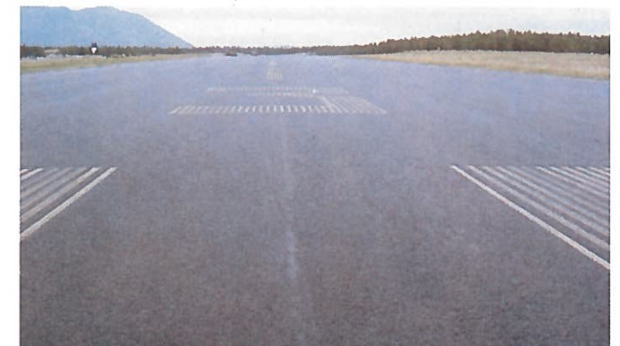
Reclamite application at this airport was completed in about one hour, and the stripping was left intact. The pavement's high void content—which allows fast water shedding in moist areas—eliminated the need for sanding after the application of Reclamite.
